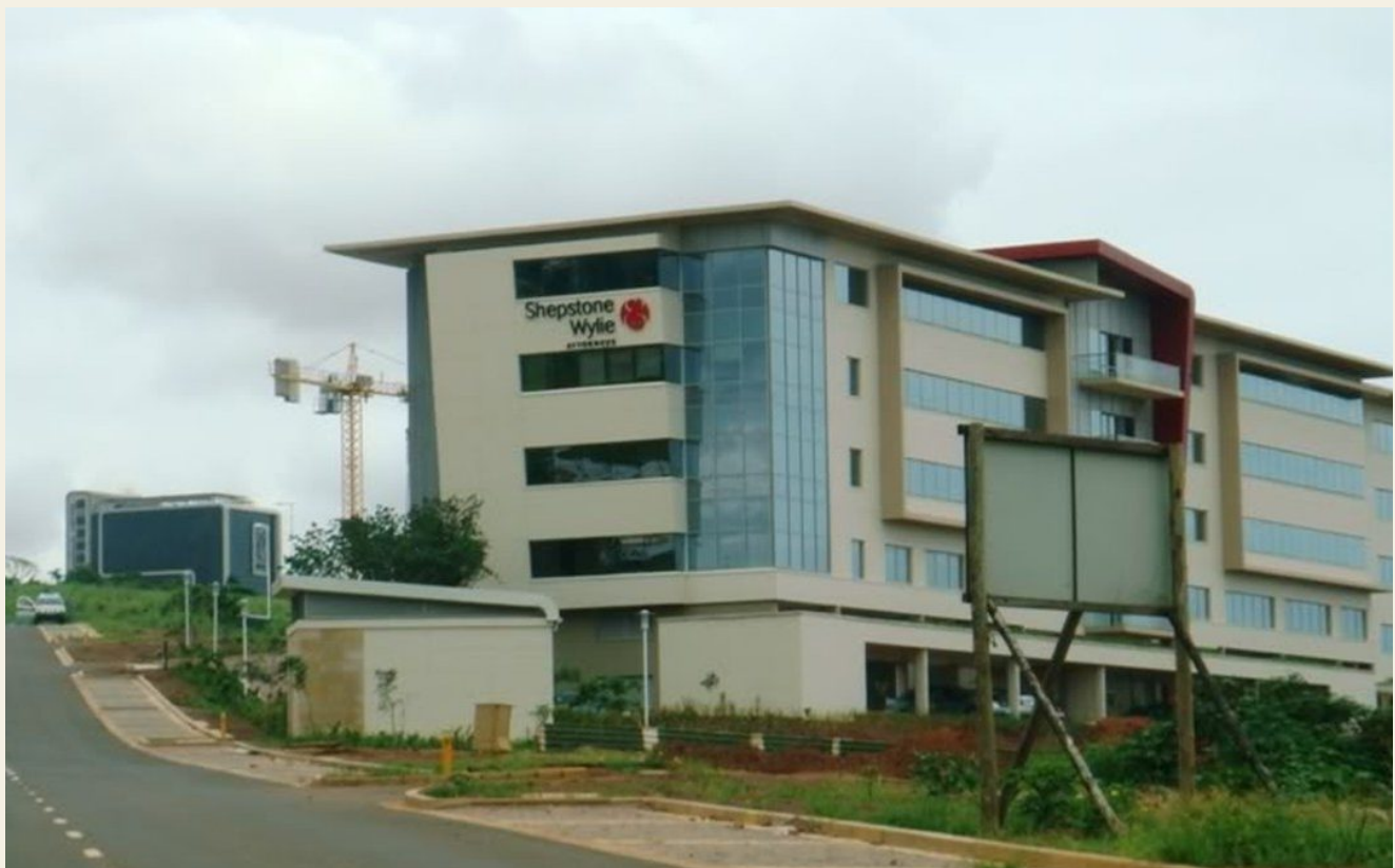
SHEPSTONE & WYLIE HEAD OFFICE
