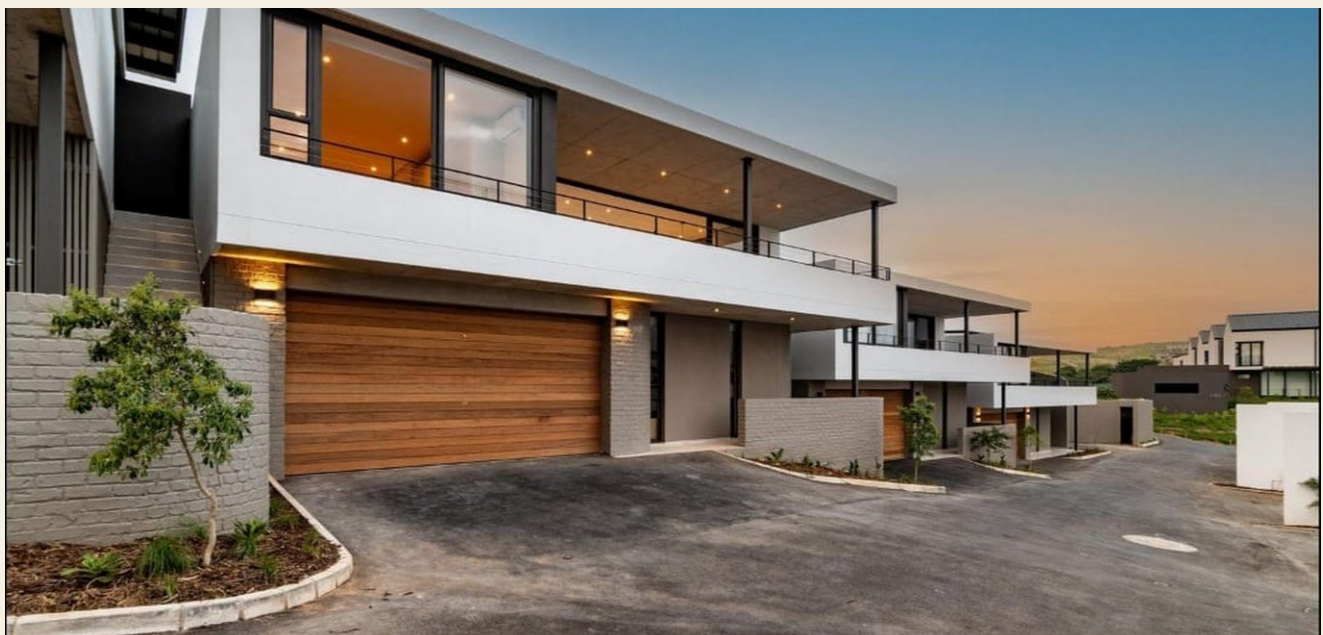
COMPLETED VALLEY VIEWS RESIDENCES
